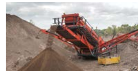
Massive stockpiling capabilities
